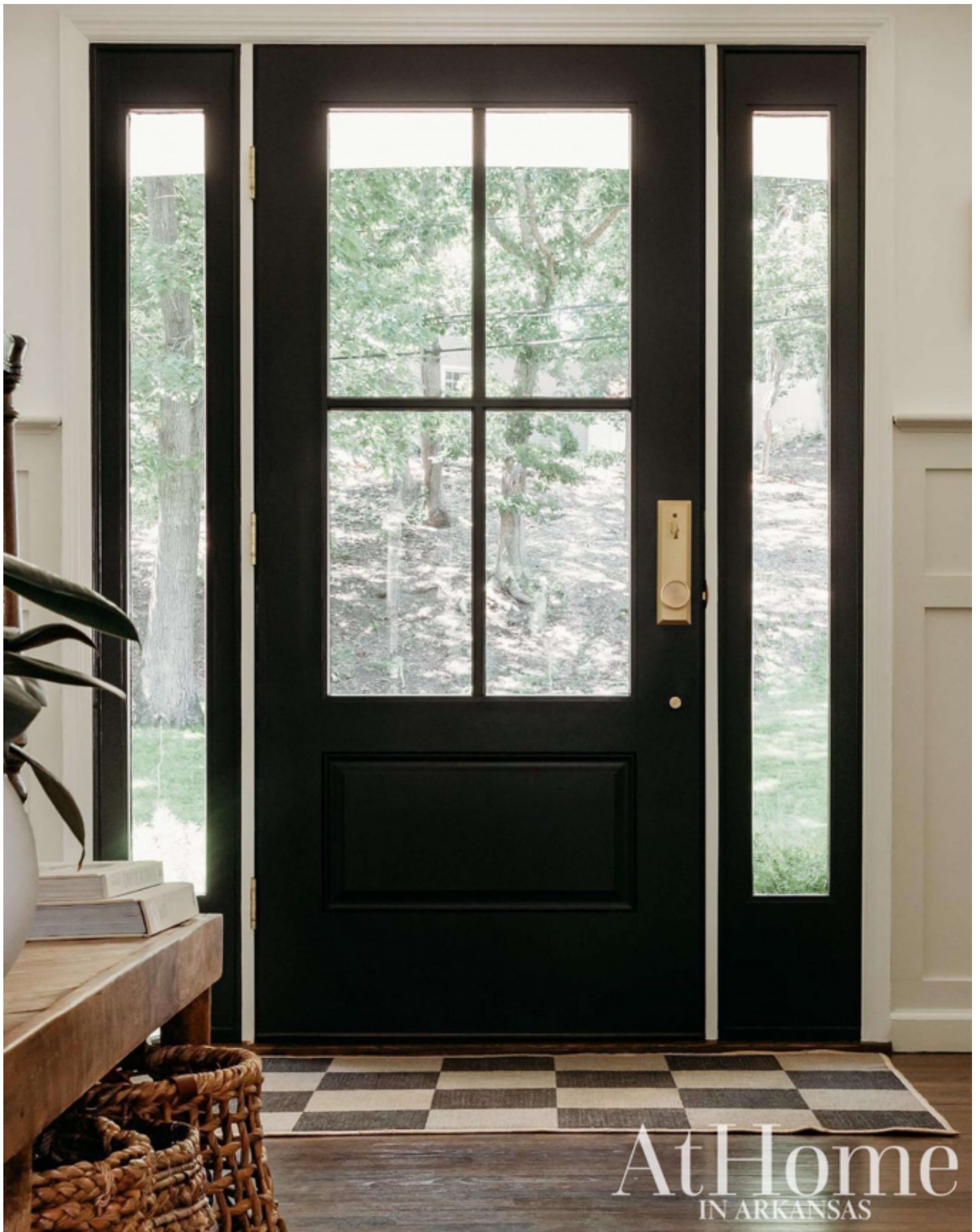
Therma-Tru "Smooth-Star" 3/4-lite, one-panel door and full-length sidelite windows, both in Onyx.
