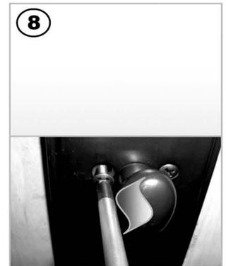
Use 1.7/16" cone-point screws to secure cylinder housing, Use of drafting or similar low tack tape will prevent marking thumb piece when tightening cylinder fixing screws.
