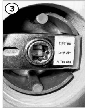
Viewed from the inside of the door the central spindle housing and the spindle are correctly located as shown.. On solid brass trim the temporary fixing of screw cover may assist in holding the grip set in position, see *figure 10*.
