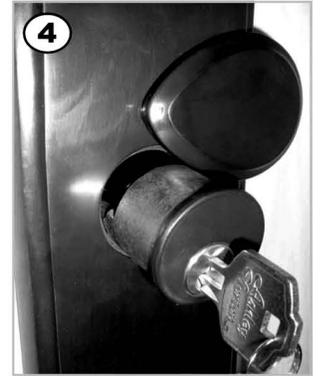
Insert the cylinder housing with the tail piece in the vertical position and then guide the tail piece and mounting posts through the deadbolt body.
