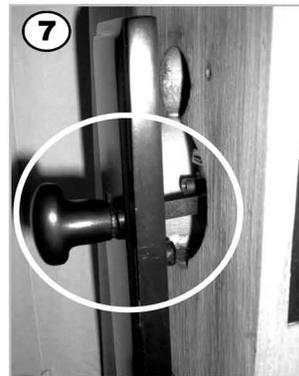
Check Deadbolt is in the un-locked position then offer up inside escutcheon locating both lever spindle and thumb piece. *Thumb piece must be in the vertical position, as shown, for correct orientation of the thumb piece.*
