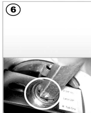
The inside lever spindle may already be pre-fitted to the inside lever, if so proceed to *figure 7*. Otherwise locate the lever spindle with the crimped end locating into the latch hub on the inside of the door.
