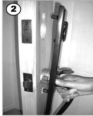
Take the exterior grip set assembly and offer up to the door ensuring that the fixing posts, the central housing and spindle are all correctly located, then push the grip set flush with the door panel.
